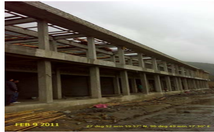
C/o Market Complex at Hawaii - Work in Progress (4)
