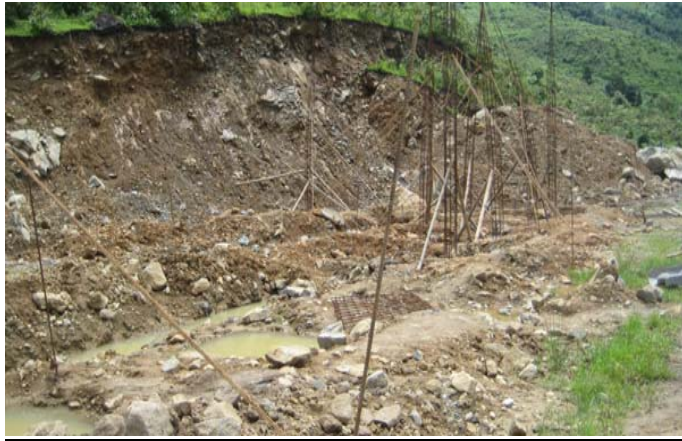
Site Preparation of Market Complex at Hawaii (1)
