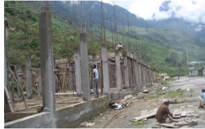
C/o Market Complex at Hawaii (2) - Work in progress
