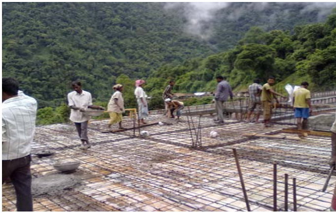
C/o Market Complex at Hawaii - Work in Progress (3)
